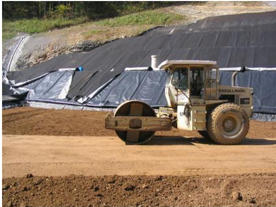
Roller Compaction
